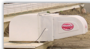
Shown: Polystainless exhaust fan with poly weather hood and pit transition hood
